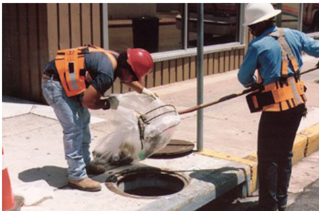
Stormwater Department crew cleaning a storm drain
